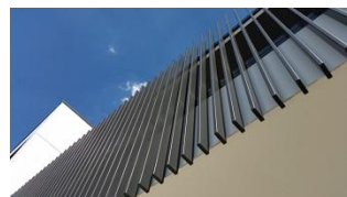
ALS# EXAMPLES OF SUNPROTECTION SCREENS: ALUMINIUM LOUVRE SCREENS WHITE VERTICAL (ALS01) AND DARK GREY VERTICAL (ALS02)
