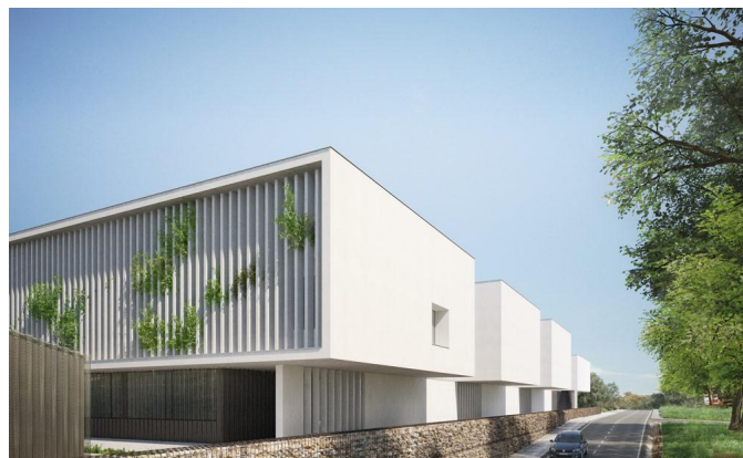
ALS# EXAMPLES OF SUNPROTECTION SCREENS: ALUMINIUM LOUVRE SCREENS WHITE VERTICAL (ALS01) AND DARK GREY VERTICAL (ALS02)
